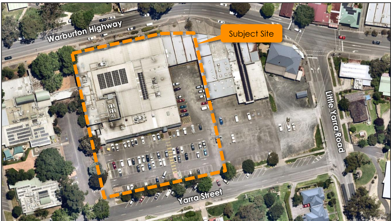
Figure 8 2450 – 2460 Warburton Highway, Yarra Junction Off-Street Parking
